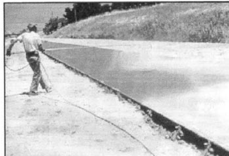
Application of liquid membrane-forming compound with hand sprayer.
